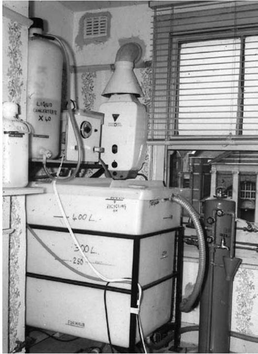
Figure 12: An example of home haemodialysis equipment, c. 1965: with Cambridge pressure and heat monitors, a tank system for dialysate, water softener and liquid concentrate, sterilized with formalin.
